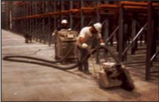
Joint preparation (cleaning) is critical in ensuring long term filler durability. The use of dry-cut type, vacuum equipped saws to clean joints is the preferred method of preparation.
