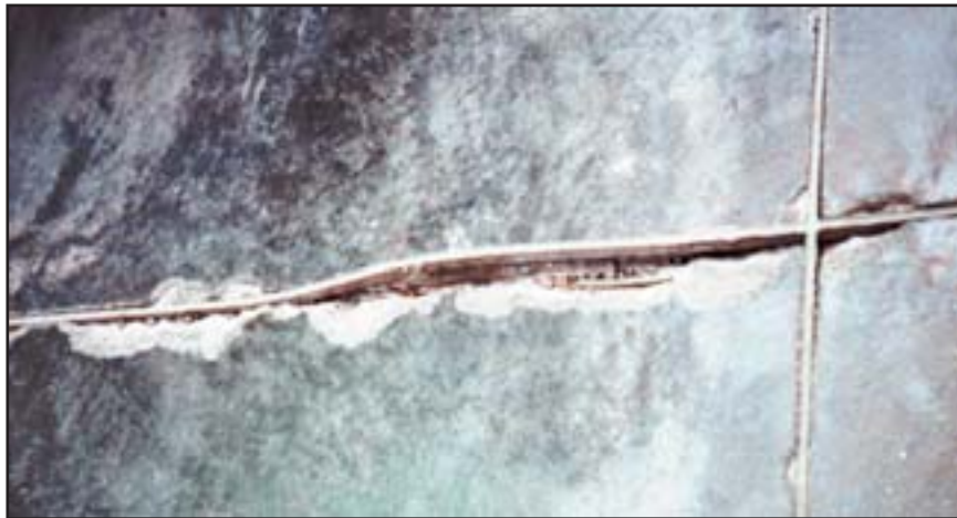
Improper filling of joints (in this case inadequate filler depth) is just one of many common causes of joint problems an owner may face, but it is one of the most easily preventable.
