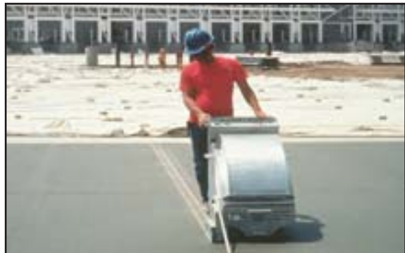
“Early Entry” saws allow for joint cutting to be performed within hours of slab placement, reducing the potential of random cracking and allowing for a shallower joint depth to induce cracking below the joint.
