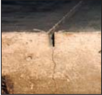
Adequate load transfer may be achieved at contraction joints if joint spacing is reduced to keep the shrinkage crack below the saw cut at 0.035" (0.9 mm) or less in width, but the effectiveness can vary.
