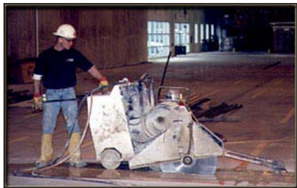
Traditional “wet cut” saws require sufficient slab cure to support the saw’s weight.
