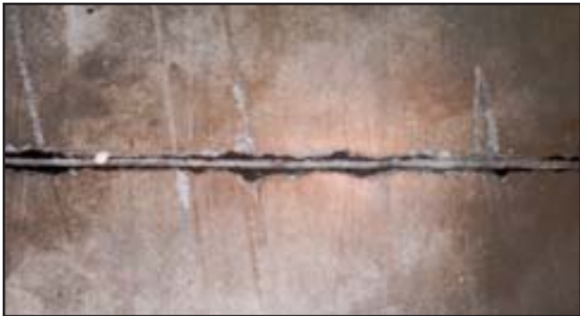
If joint filler has dropped below the floor surface or was not flush originally, joint edge spalling may occur.
