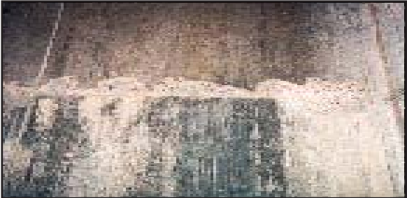
In theory, all joint edges likely suffer from some degree of curl. Whether the curl is significant or not is determined by whether it interferes with the material handling operations and leads to joint edge deterioration.
